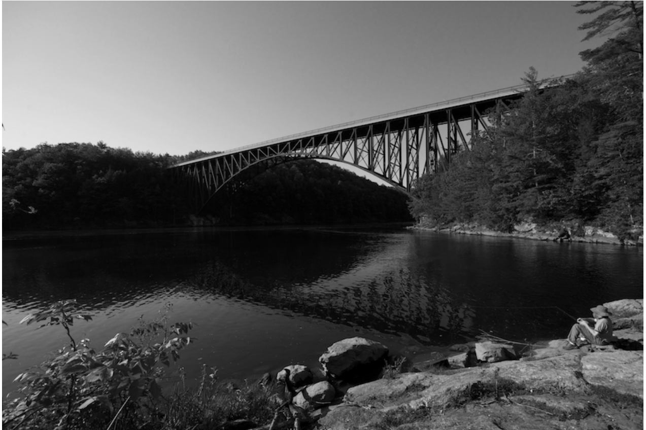
French King Bridge Over Connecticut River - Erving
